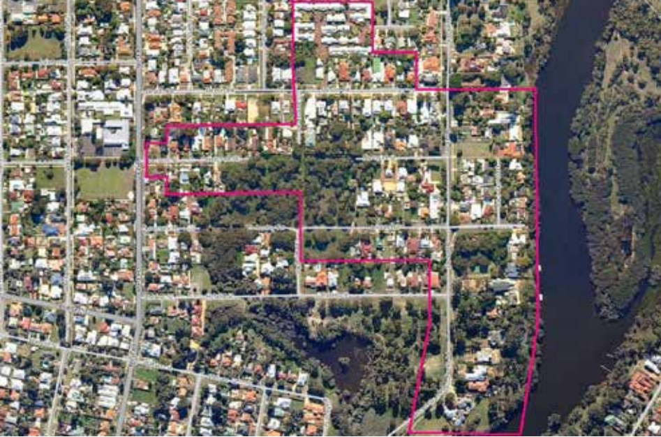
Image 3-K: Anstey transformer LV network
